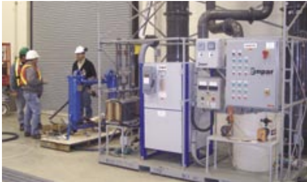
Technicians install ENPAR pilot project.
